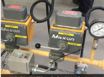
Gas Safety Shut-Off System Pipe Train With Leak Detector.
