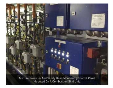
water gauge (1 millibar) to operate and shut-off the gas supply to the mixer with the solenoid valve if the manifold mixture pressure falls below 0.5 inches water gauge (1.25 millibar) further preventing a backfire from occurring. The cause of the low manifold mixture pressure would still then require investigation and could be due to a leak in the mixture pipe work or burners or incorrect setting of the mixer minimum physical stop screw.
