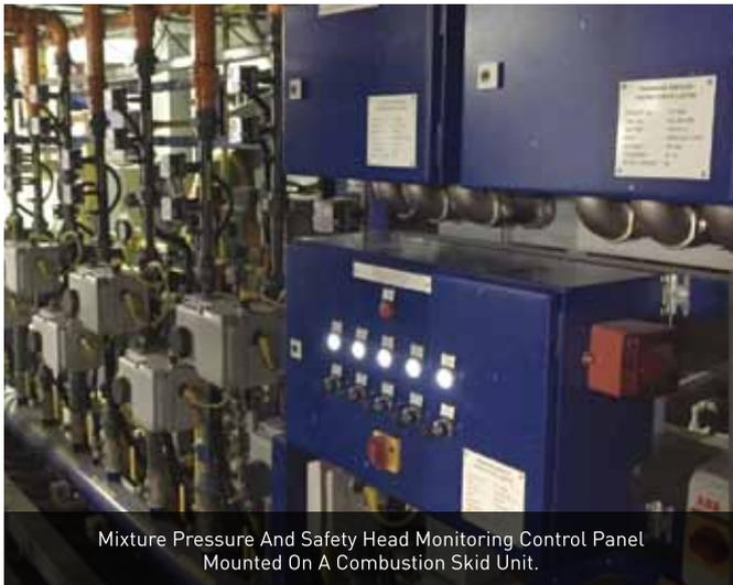
Mixture Pressure And Safety Head Monitoring Control Panel Mounted On A Combustion Skid Unit.
